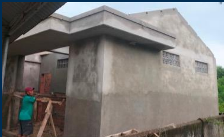
The completed exterior awaiting finishing and painting.
